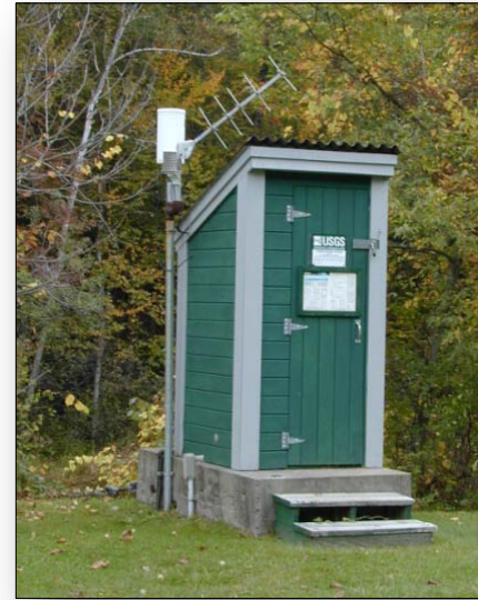
Figure 5. USGS cooperative stream gage at USACE Union Village Dam, Thetford, VT (Gage # 0114500, Ompompanoosuc River at Union Village, VT). (Photo courtesy USACE New England District).
